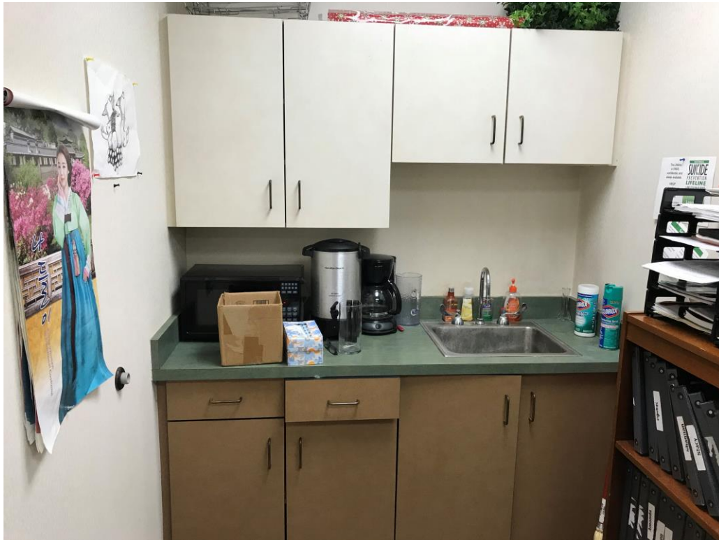
Existing Cabinet and Countertop
