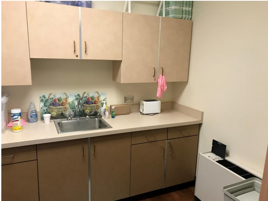
Existing Cabinet and Countertop
