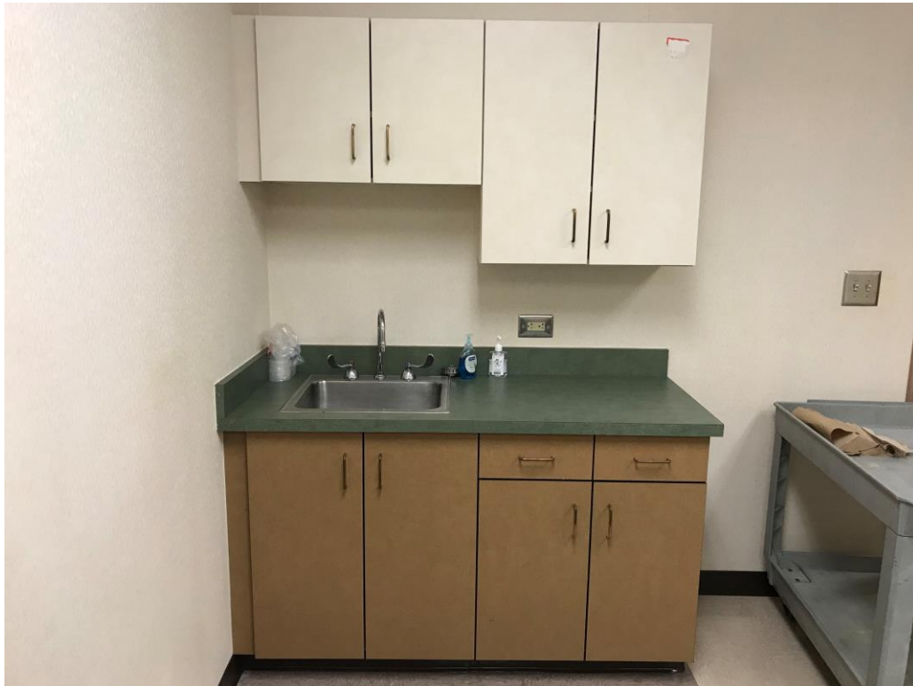
Existing Cabinet and Countertop
