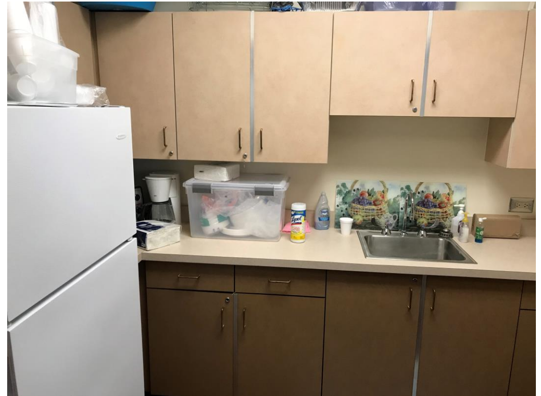
Existing Cabinet and Countertop
