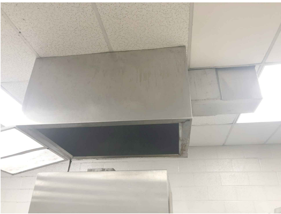
B EXISTING EXHAUST HOOD & EXPOSED DUCT NTS
