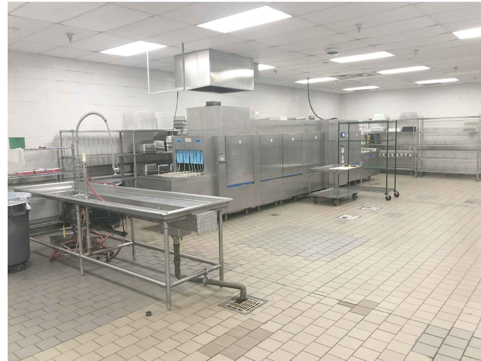
B DISH MACHINE AND HOOD NTS
