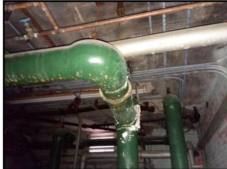
12 The hard joint insulation over the sulfur rock insulation tested positive for asbestos (2% Chrysotile).
