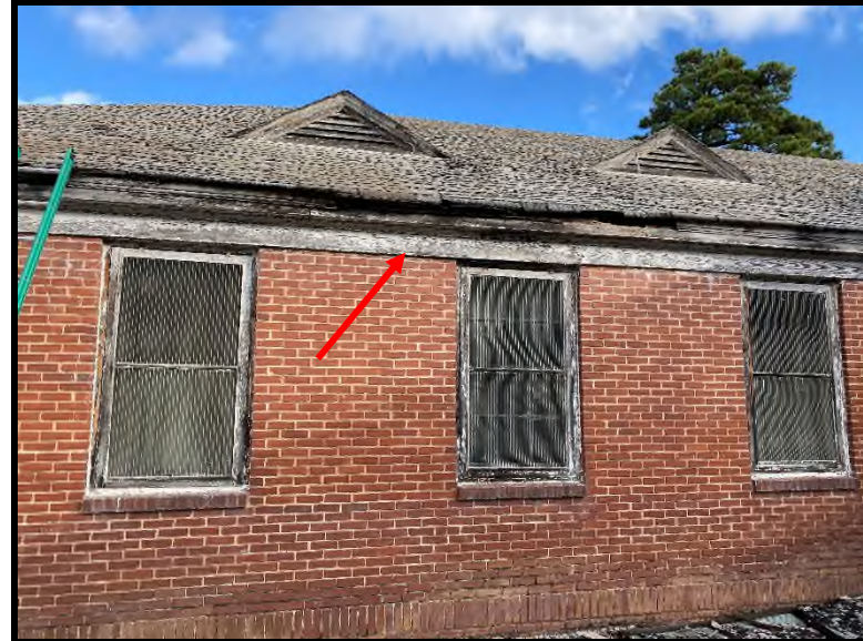
10 The white fascia board tested positive for lead-based paint (6.4 mg/cm 2 ).
