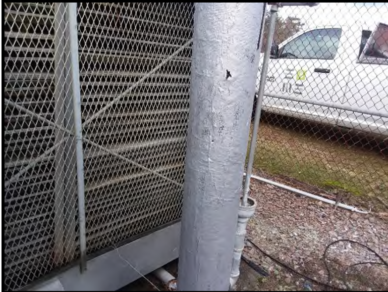
5 The pipe wrap on the sulfur rock insulation tested positive for asbestos (6% chrysotile).
