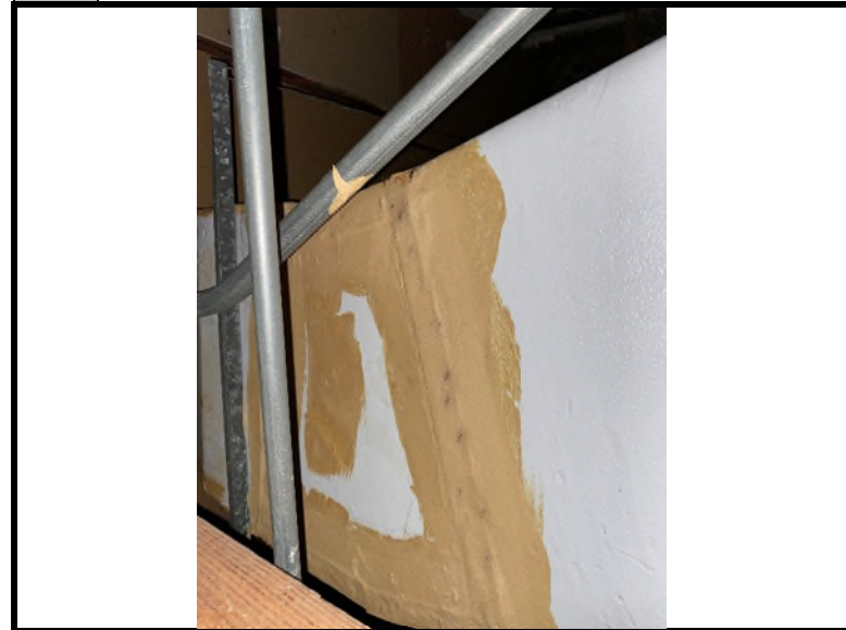
8 The yellow duct mastic located on the HVAC ducts tested positive for asbestos (5% chrysotile).
