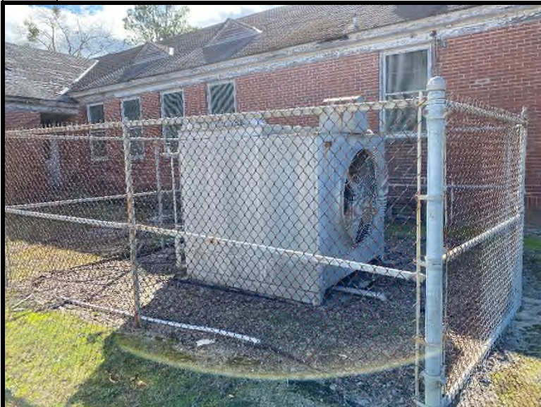
3 The silver paint located on the cooling tower tested positive for asbestos (3% chrysotile).
