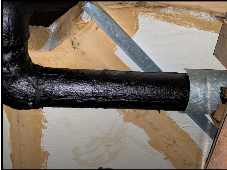
9 The black pipe mastic located in the building tested positive for asbestos (5% chrysotile).
