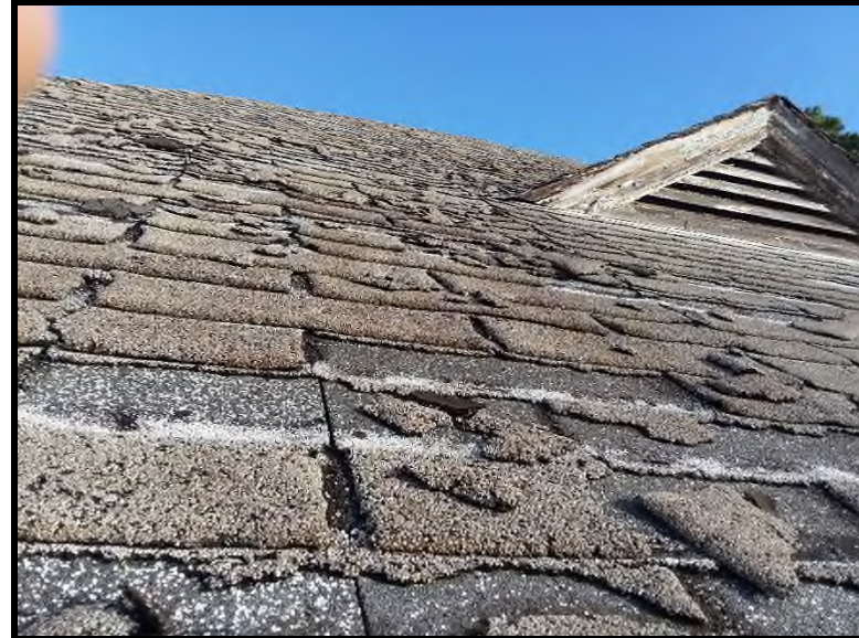
2 The asphalt shingles tested positive for asbestos (2% chrysotile).
