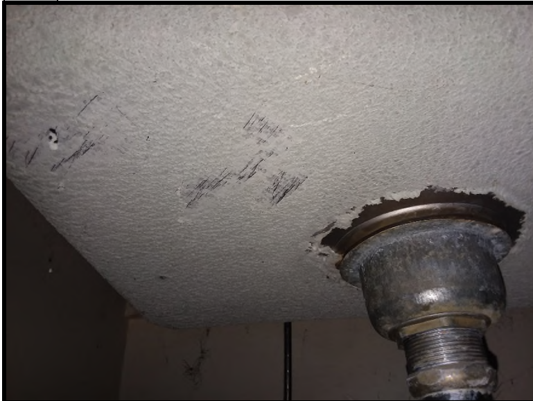
7 The gray sink coating located on the south side of the building tested positive for asbestos (4% chrysotile).
