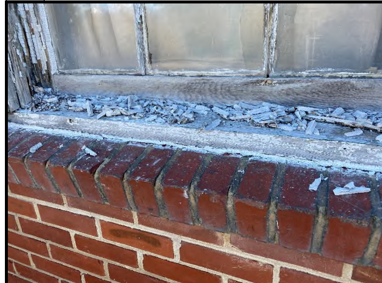
4 The exterior window glazing tested positive for asbestos (2% chrysotile).
